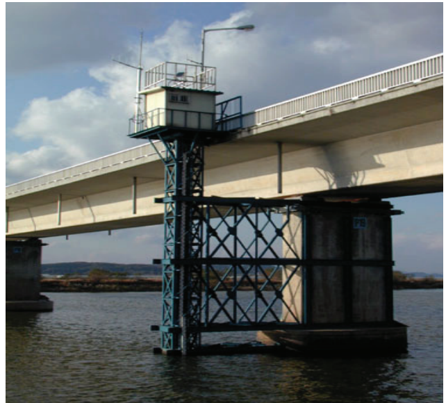
Fig. 4-2 Float gauge (with stilling well)
