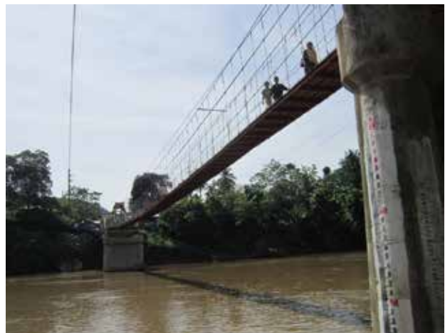
Fig. 11 - Hanging footbridge constructed after the destruction of the Bridge (Cabula-Maasin, Bukidnon province)
