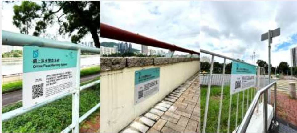
Figure 30 – QR code installations at the riverside and the subways' entrances.
